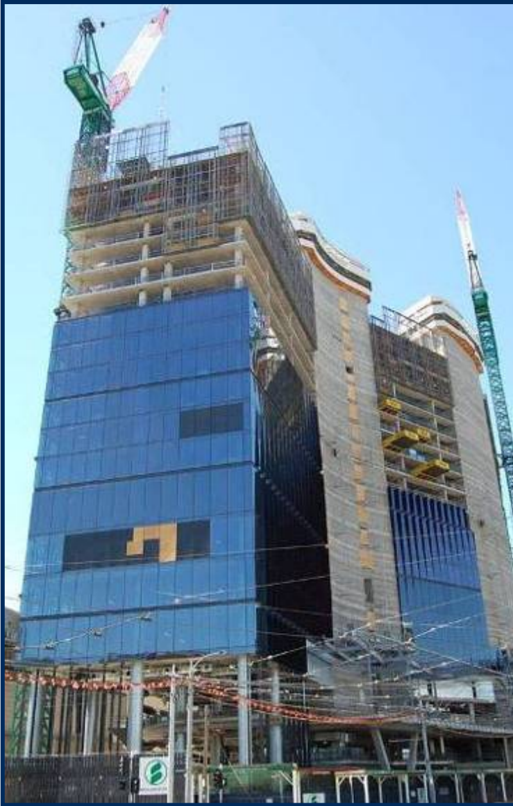
Construction of Third Hotel
